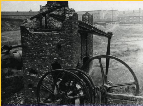
▲ FIGURE 11-1 JAMES WATT'S STEAM ENGINE This Watt steam engine in Wolverhampton, England. Steam injected in a cylinder (inside the brick housing) pushes a piston attached to a crankshaft that drives machinery (right side of engine).
